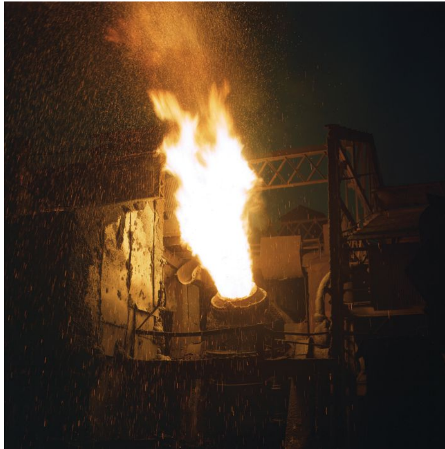
A scene in a steel mill, Republic Steel, Youngstown, Ohio. Molten iron is blown in an Eastern Bessemer converter to change it to steel for war essentials. Photo Credit: Alfred T. Palmer, 1941, Library of Congress
